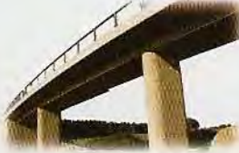
a concrete bridge
